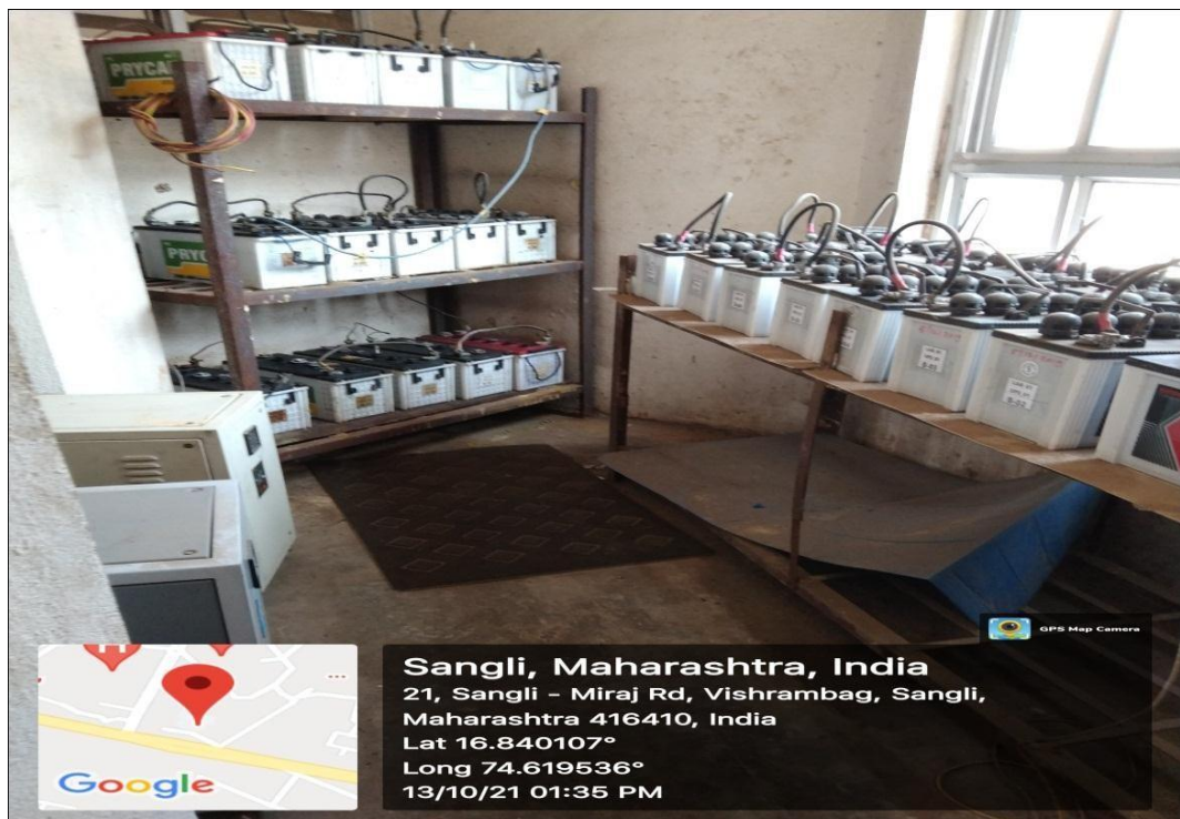
Set of Batteries used for Power backup at VPIMSR.
